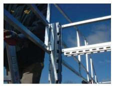
STEP 7 Install the centre truss (has 3 angled tubes welded on each side). Lift it to the top of the peak and slip each end into the sockets on the inside of each peak truss.
