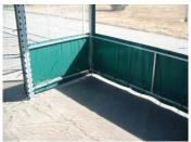
Once all tywraps are in place, tighten them starting with the ones in each corner, then the ones in the centre of each side working your way outwards. Repeat this step for all sides until the vinyl is snug to the frame.
