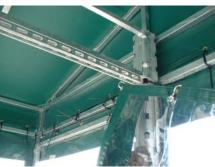
Insert the Velcro tabs through the "D" rings up one side. Pull the curtain snug and insert the Velcro tabs through the "D" rings on the other side.
