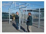
STEP 9 Lay out the two side panels (8'9"x8'8") on the ground on either end of the peak trusses. Insert the adjustable feet in each corner and fasten in place with a bolt threaded into the welded-on nut.
