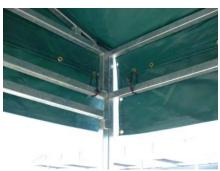
STEP 16 Install tywraps loosely into all remaining grommets around the perimeter, starting with each corner, then working out from the centre of each side. Tighten the tywraps, starting with each corner, then working out from the centre of each side, until the vinyl in snug on the structure.
