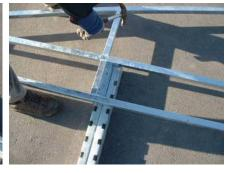
STEP 3 **IMPORTANT:** Install the "J" locking pins through the bracket into the post. Make sure they sit so that the head is flush with the bracket.
