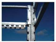
Install the 2nd peak truss. Lift to the top of the outer posts. Position the truss so that the "hooks" on the bracket sit into the slots in the post. Tap the brackets with a hammer to ensure they are in place. Install the "J" locking pins.
