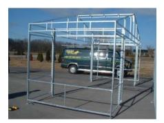
Lay out the 6 purlins. One at a time, slide one end of the purlin into the angled tube on the top centre truss and position the other end so that the "U" bracket sits over the top of the side wall panel. Repeat this step for all 6 purlins. Check that they are straight and parallel to the front and back peak trusses. Insert bolts and tighten with nuts.
