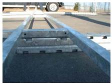
STEP 4 Lay out 1 post and 1 - Truss w/ Track. Position the truss so that the "hooks" on the bracket sit into the slots in the post. Tap the brackets with a hammer to ensure they are in place. Install the "J" locking pins. Repeat for the second set.
